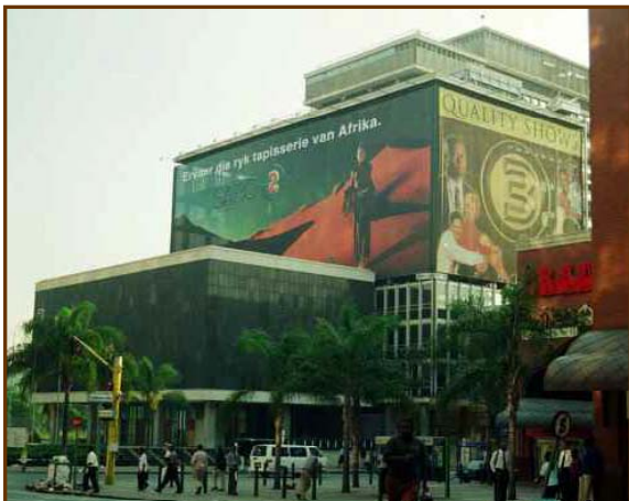
Huge computerized advertising panels concealing burned out floors of Munitoria
