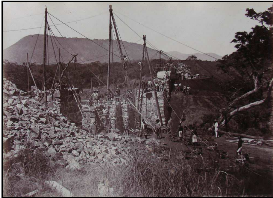
A contemporary photograph, showing the construction of one of the bridges during the building of the railway line in the 1880s
