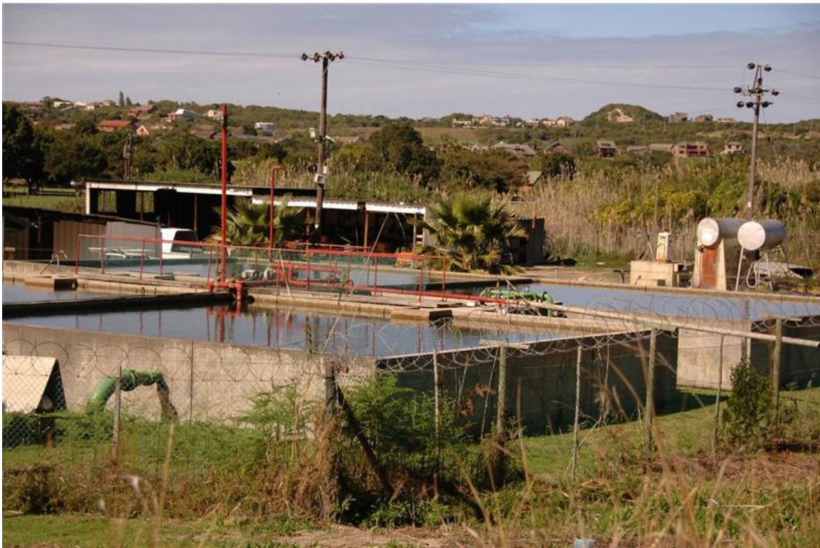
Photo: Water purification plant near Wilderness
