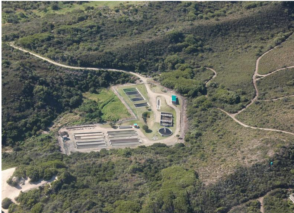
Photo: Kleinkrans water treatment plant
