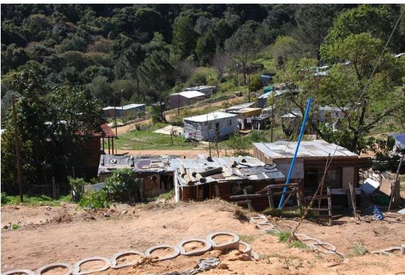
Photo: development on steep slopes
