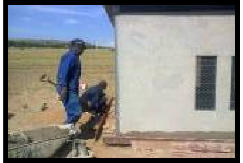
MOKWETE PUMP HOUSE
