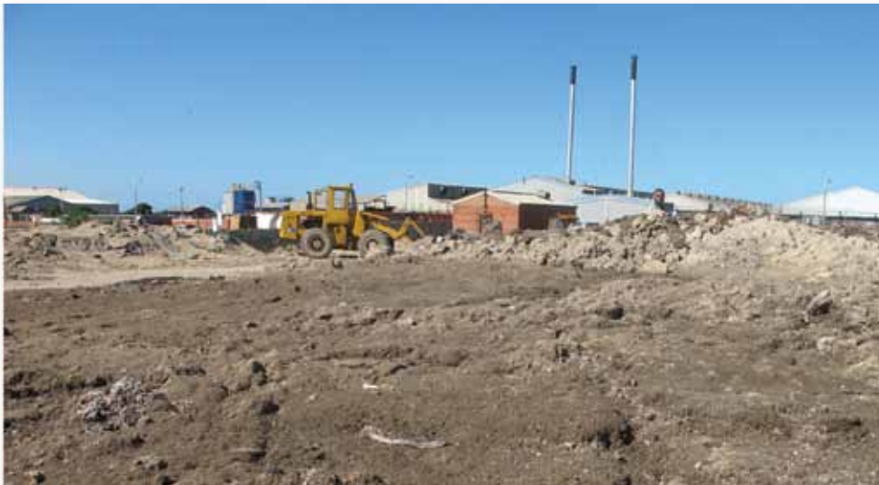
Decommissioning of unlawful waste disposal facility in process
