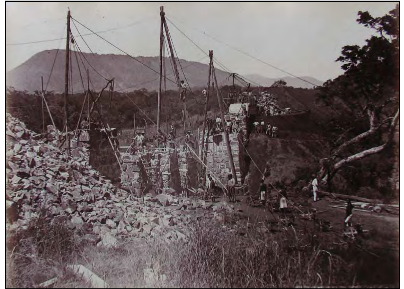
A contemporary photograph, showing the construction of one of the bridges during the building of the railway line in the 1880s
