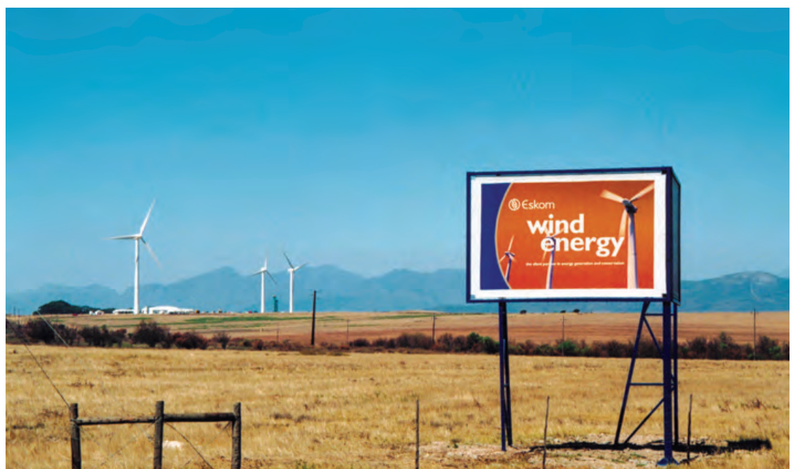
An Eskom wind trial plant, experimenting towards renewable energy for future use. Photography: Eskom
