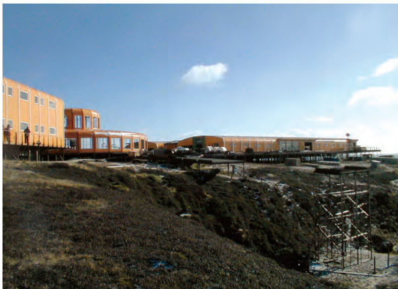
Marion base under construction. Photography: Adriaan Dreyer
