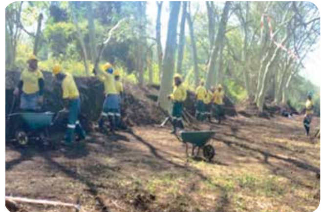
Above: One of the Maputaland Project teams removing an artificial earthen berm from the bank of the Mkhuzi River
