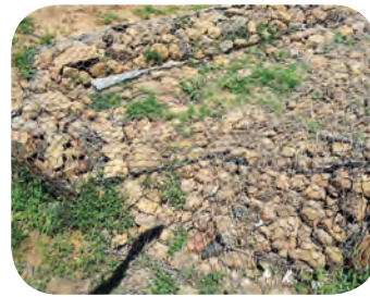
Above: After rehabilitation.
