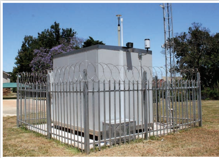
A monitoring station which houses special instruments to measure air pollutants.
