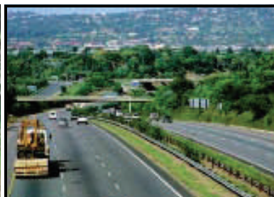
Transportation: Freeway, Pretoria
