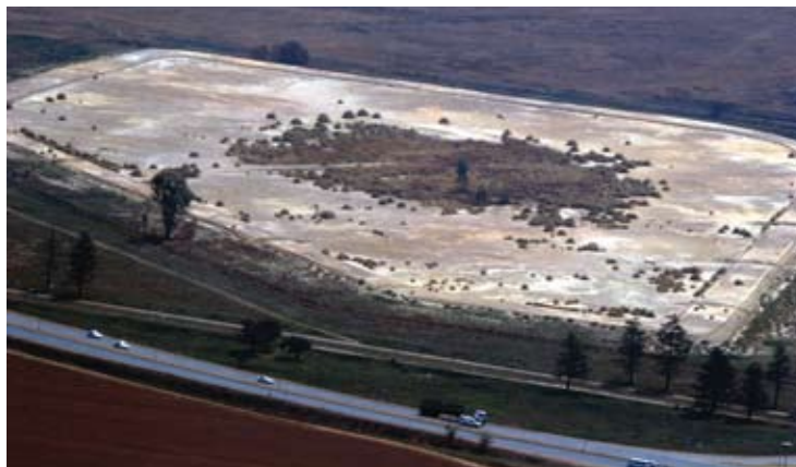
A mine tailings dam along the Johannesburg gold reef.
