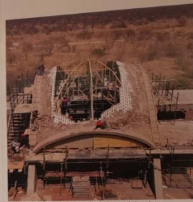
Construction of vault with formwork in place
