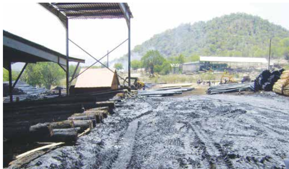
Processing area: Contaminated soil due to it being unlined
