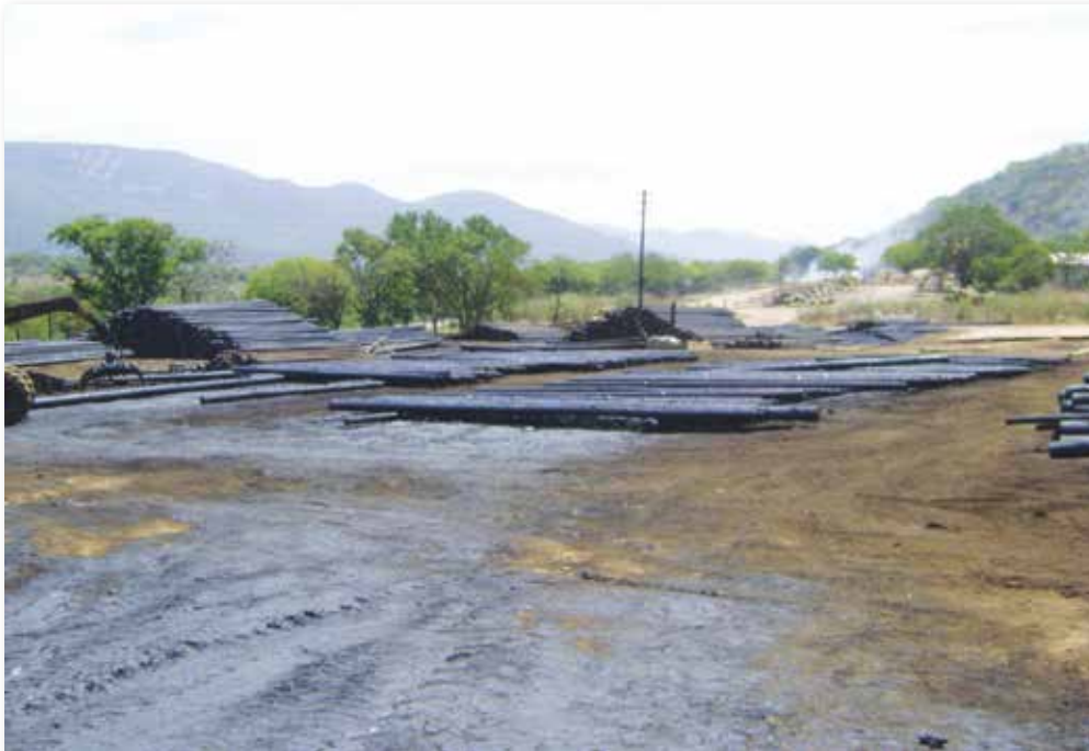
Contaminated soil in the vicinity of the CCA Plant
