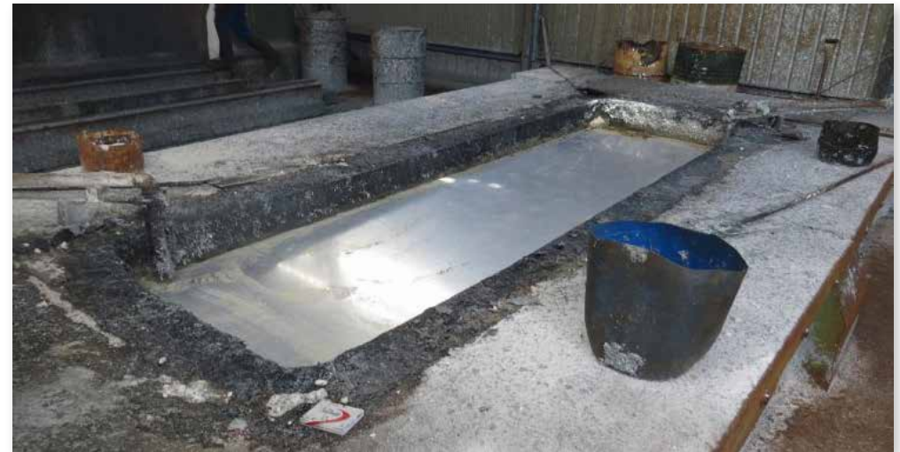
Picture: Hot Dip Galvanising
