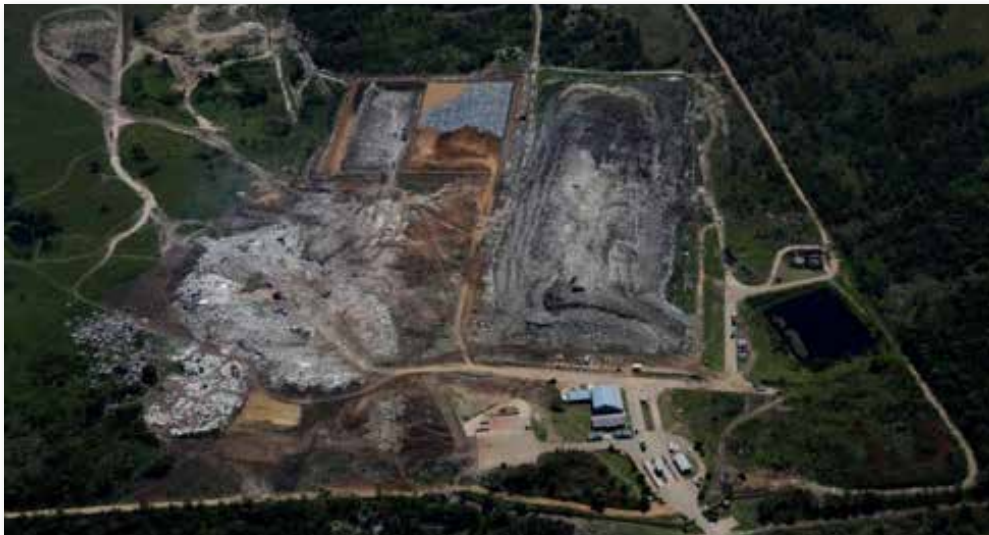
Picture: Uncovered, uncontained, uncontrolled.
