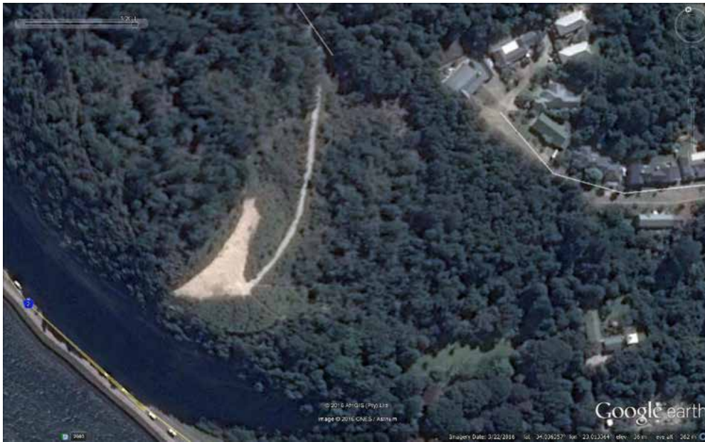
Picture: After notice was issued: March 2016. Stable platform, well-vegetated with stable flanks.
