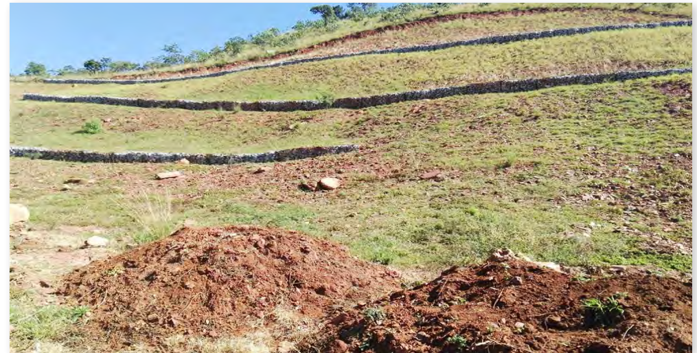
Hilltop 1: After Rehabilitation
