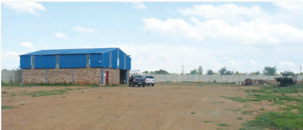
Warehouse where health care risk waste had been stored
